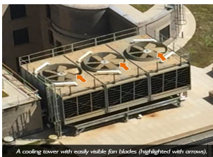
A cooling tower with easily visible fan blades (highlighted with arrows).
